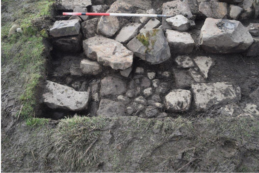
The gap in the cross-wall, looking west. The 1m ranging pole is placed across the gap. The rubble blocking the gap is still in place under the pole. In the rubble are some long (0.7m) flat stones which may have been lintels (see discussion section).
